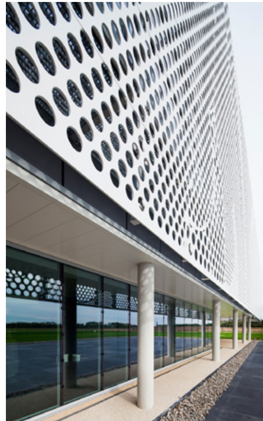
Creation: PAD Architectes for BERI 21 | Fabrication: LCCA | Photo: Mathieu Ducros
